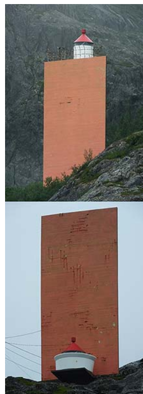
Jakobselv Range Lights Forward Range Light (bottom)—Rear Range Light (Top)
