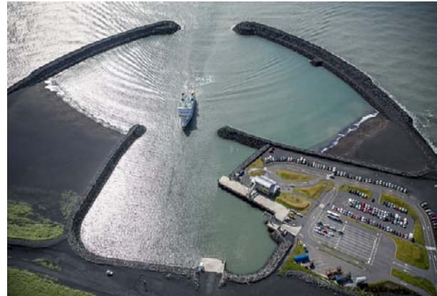
Landeyjahofn Ferry Terminal
