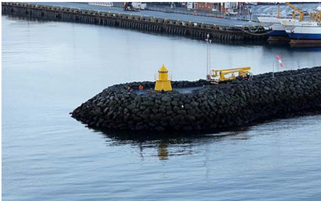
Skarfagarðs Light at Reykjavik Breakwater
